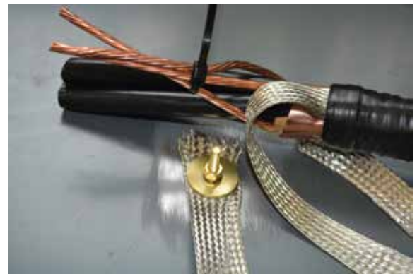
Installation Prep Photo
